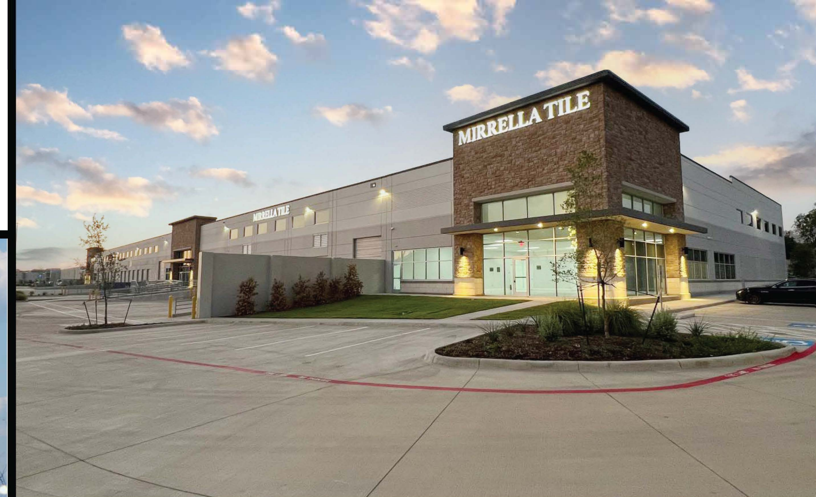
Showroom & Warehouse: 2303 E-Interstate 30. Grand Prairie, TX 75050
